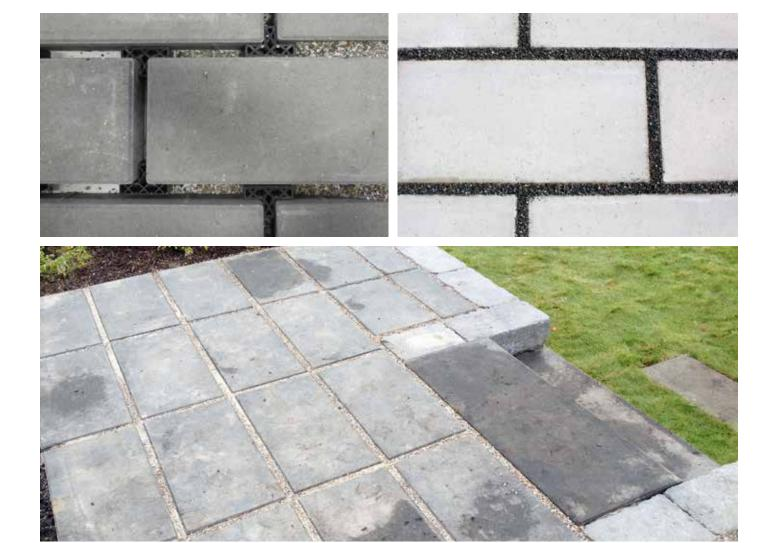
The correct solution is a combination of bottom material, slab/stone size and gap. The target is to obtain an open surface of 10-14% suitable for traffic kategori T2.
